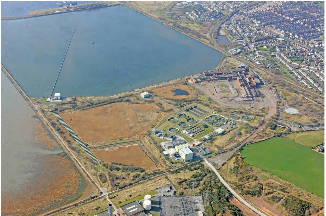
View of part of Action Plan Area looking east across Salhouse Mills and Cavendish Dock
