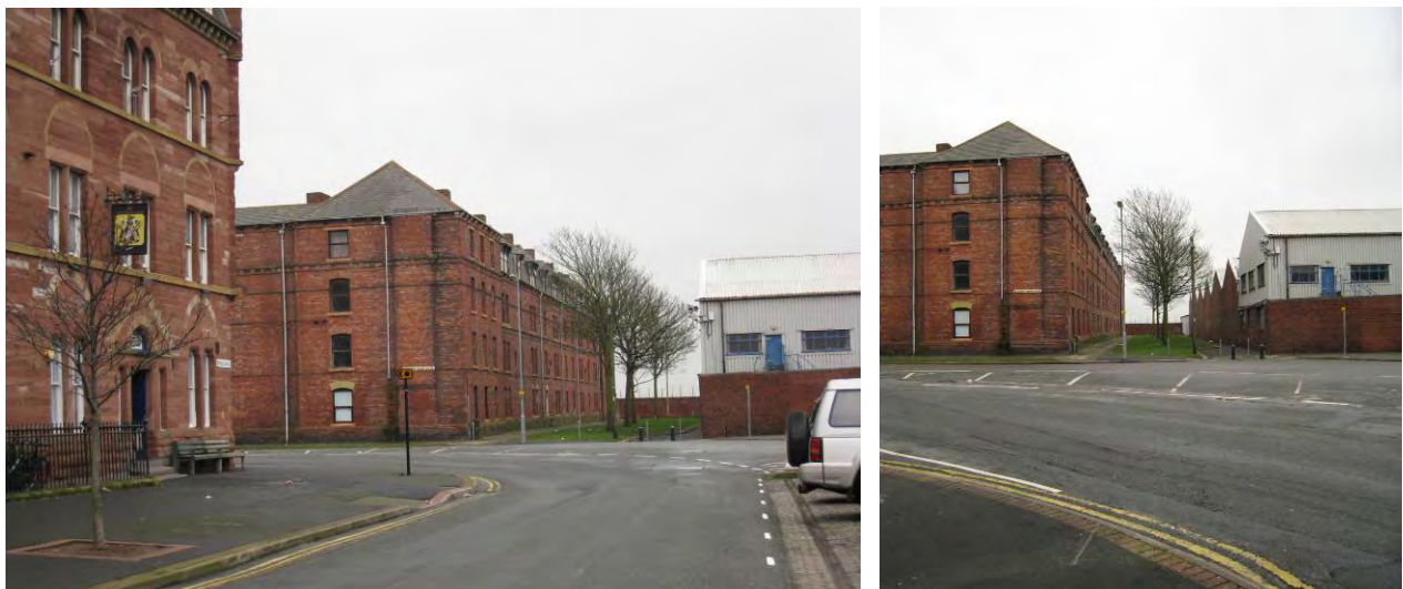
Route for the new Western Dock Access Road at Barrow Island. The buildings on the right have been removed to accommodate the new road.
