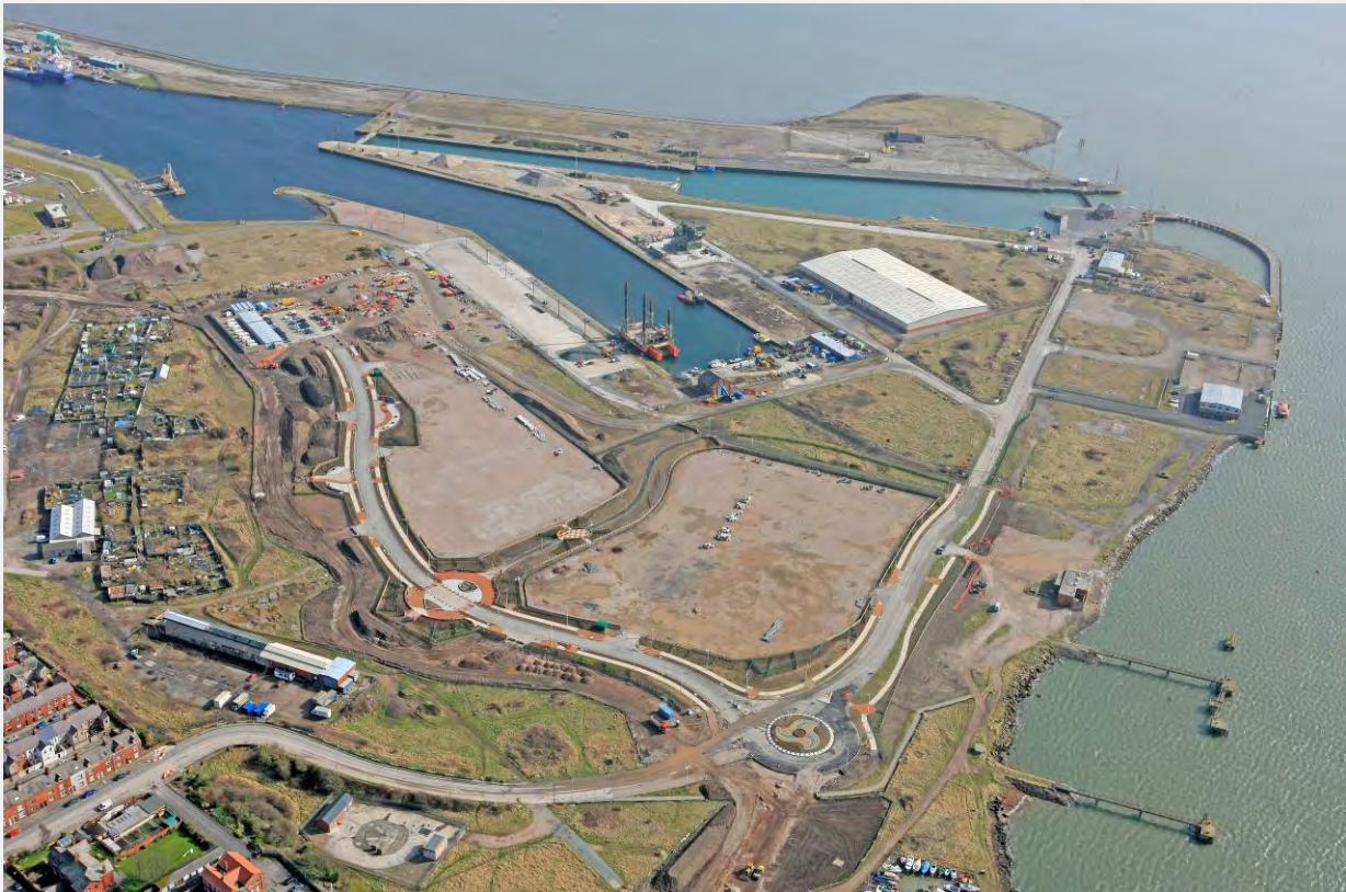
Figure 19: Aerial View of Waterfront Business Park Spine Road under construction
