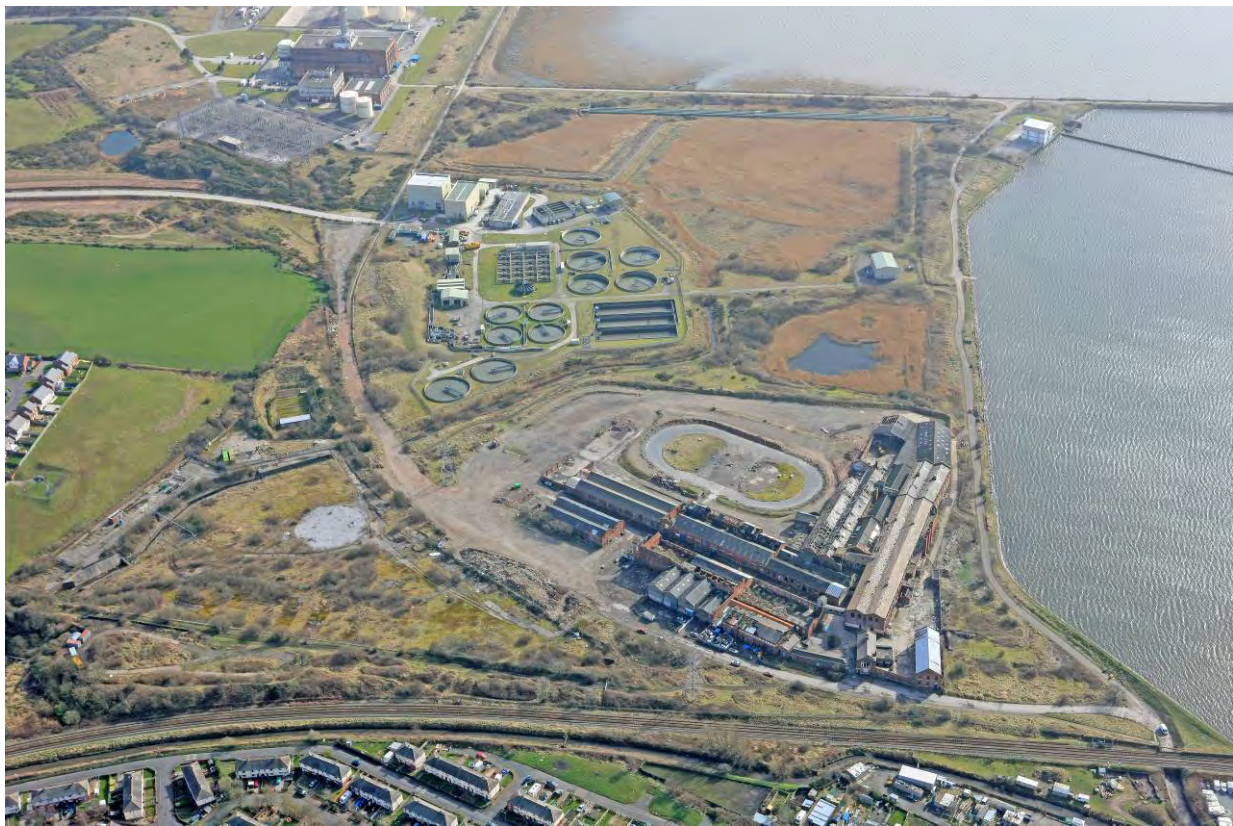
Aerial View of Salthouse Mills and the Wastewater Treatment Works
