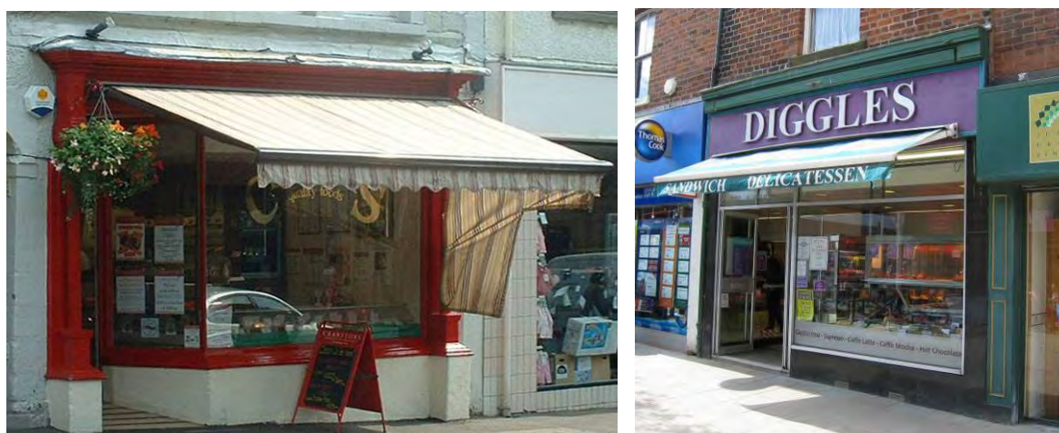
These modern retractable blinds are often suitable modern alternatives if carefully positioned. The original blind box is still in place at Diggles on the right
