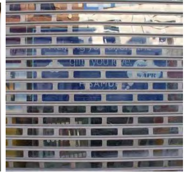
○ 'Punched' type shutter with transparent polycarbonate vision panels, normally in aluminium
