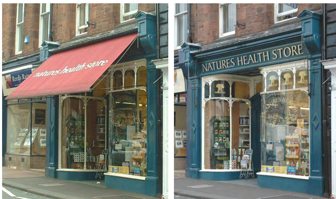
An attractive & well-maintained traditional shopfront with fully-retractable canvas blind – see also Hartley's front cover
