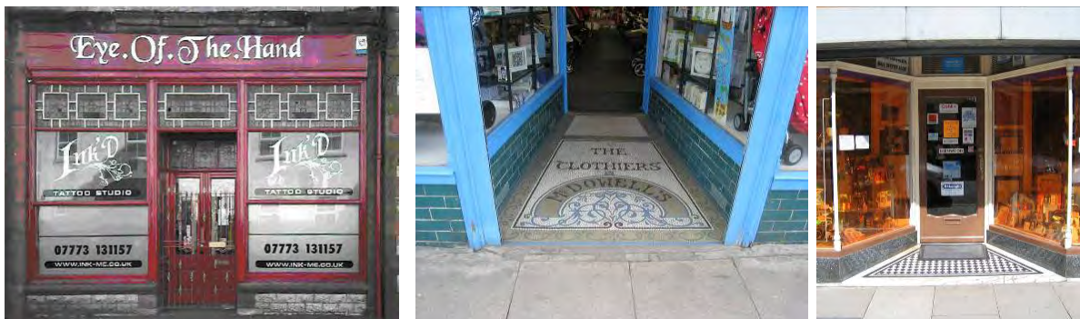
Left: Shopfront of 1892 at the former drapery department of the Co-operative store Dalton, shows the emerging Edwardian Style with stained glass clerestory lights, but with large Victorian sash shop windows. Centre: Mosaic tiled deeply recessed doorway at Baby Bitz, Cavendish Street, Barrow (the current shopfront is a replacement of an earlier even more ornate Edwardian Shopfront and dates from c1920?) Right: Edwardian/1920's style shop door at Hurleys, Cavendish Street, Barrow
