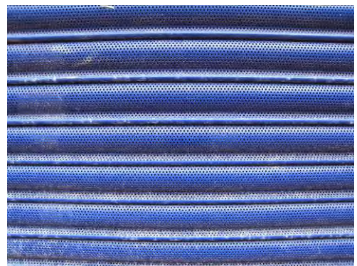
✗ Painted perforated lath type steel roller shutter
