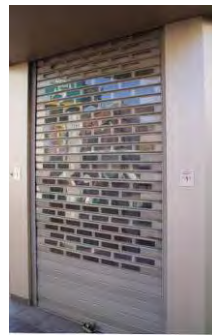
○ 'Punched' type shutter with transparent polycarbonate vision panels, normally in aluminium
