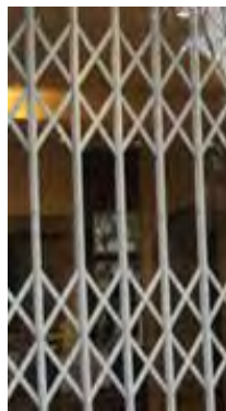
✓✓ Retractable internal lattice gate type shutters
