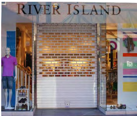
✓ Separate external doorway shutter predominantly of the punched grille type but a slimmer profile giving greater transparency
