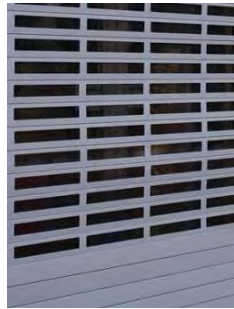
○ 'Punched' 'stamped' or 'cut' type shutter, available in aluminium, steel or plastic
