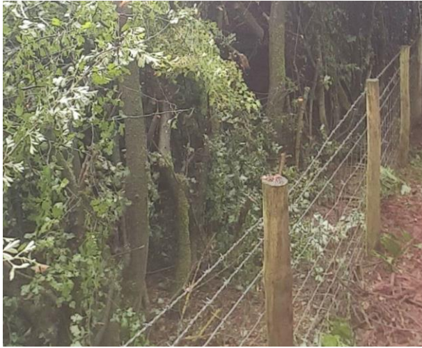
Perimeter Fence cut back in progress
