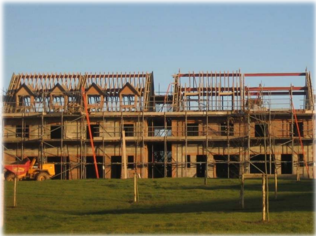
22: Housing Development, Barrow
