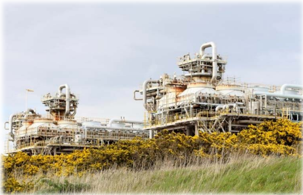
17: Gorse habitat at Barrow Gas Terminal
