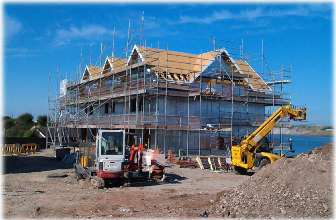
21: Housing Development, Barrow
